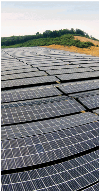
29,092 Yingli PANDA Monocrystalline 60 Cell Series Panels sit atop Hang Tuah Jaya, Melacca, Malaysia
